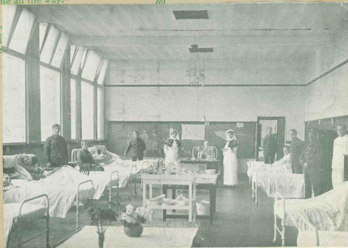
Blackboard Room as a Ward.
